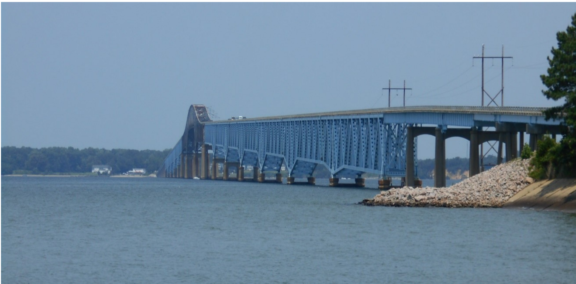
Norris Bridge over the Rappahannock
